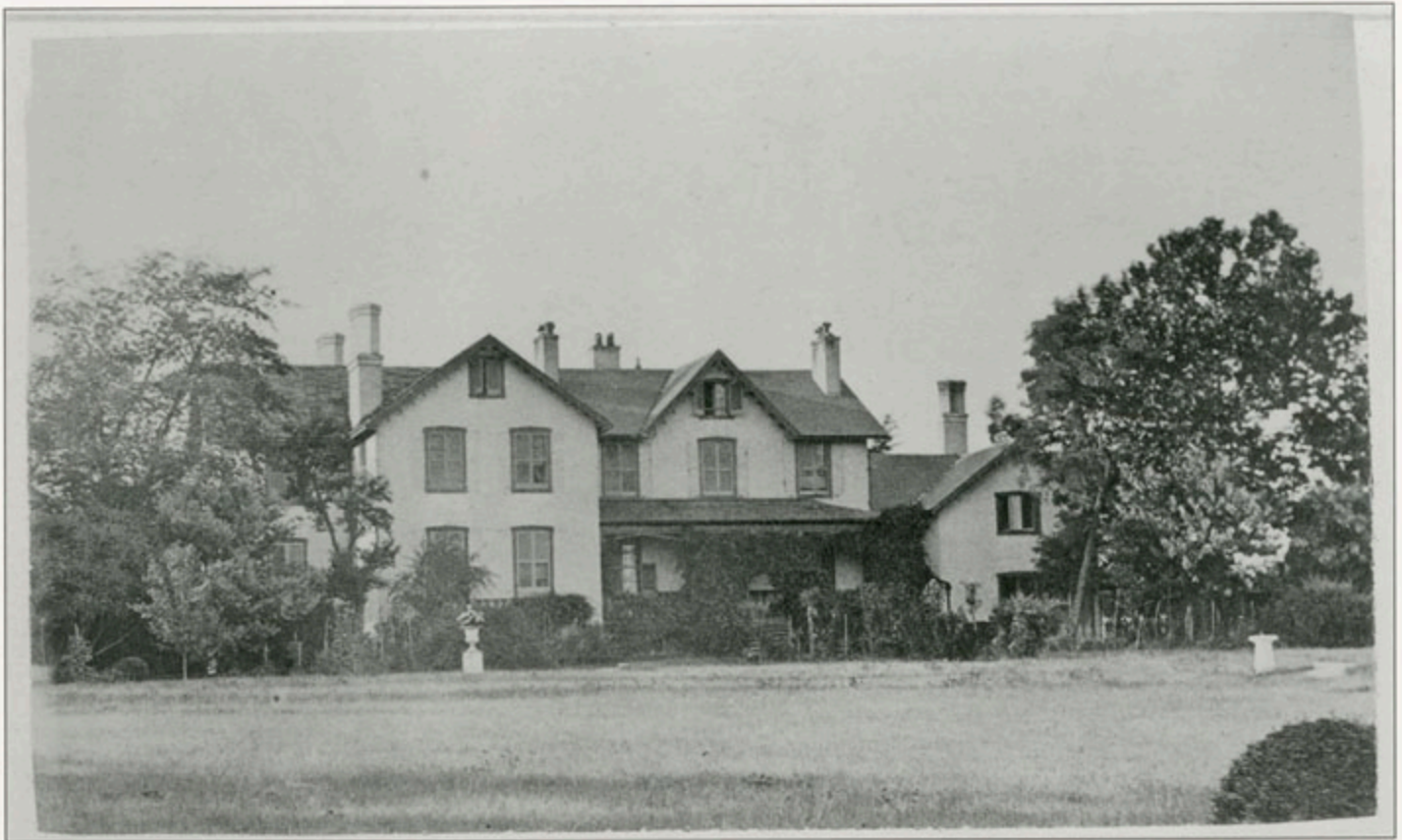
Anderson Cottage at the Soldiers' Home complex. TLM #3993
