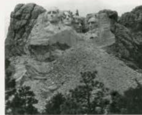
The original under construction. (TLM #1945)
