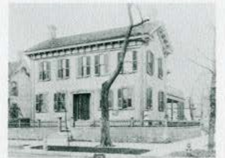
The excessive trimming of the elm tree, as indicated by this photograph, would lead one to believe that it would not have long to live.
